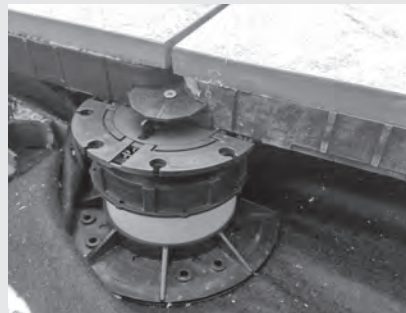
▲ Locking pedestals or fasteners may be necessary to address wind uplift and prevent paver displacement.
