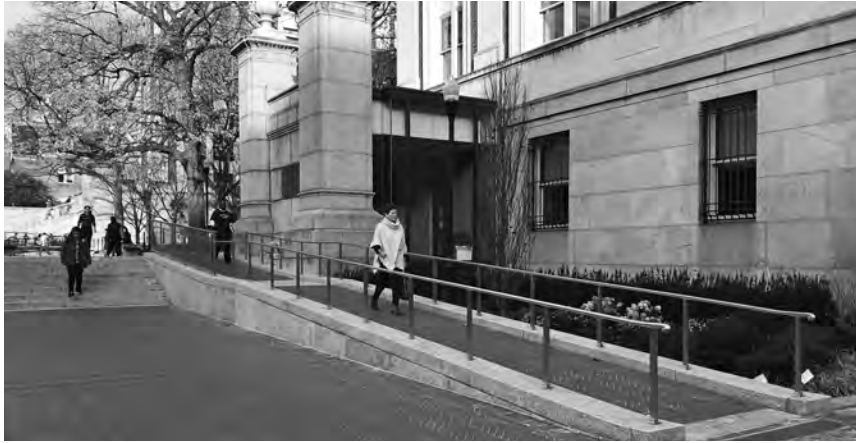
A Retrofitting ramps at historic / landmark plazas poses logistic and design challenges but is often required, both for code compliance and for universal access.
