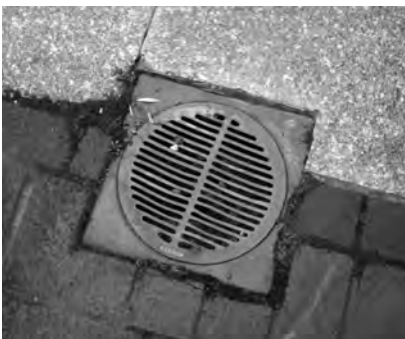
▲ Area drains provide bi-level drainage, at both surface and membrane levels.
