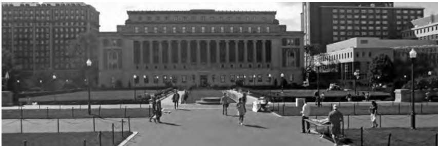
▲ Columbia University, Butler Library , New York, New York, Plaza and Hardscape Rehabilitation.
