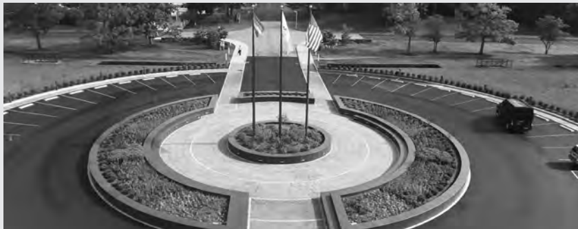
▲ Completed plaza, situated above an underground parking garage.
