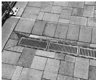
▲ Trench drains remove surface water across the entire width of a ramp or slope.
