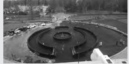
▲ Waterproofing membrane installation.
