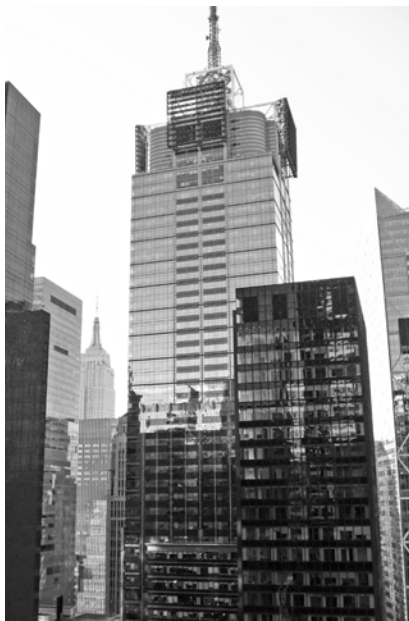
▲ What can be done to improve the performance of aging glass buildings?
