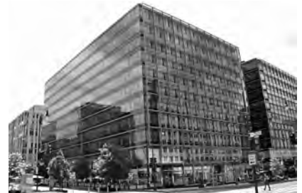
▲ CityCenterDC, Washington, District of Columbia, Facade Condition Assessment.
