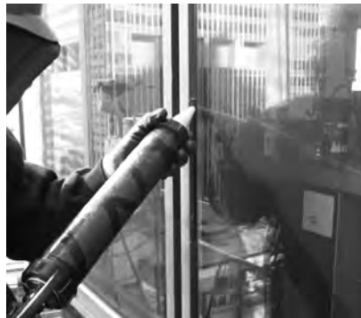
▲ Wet glazing an existing glazed curtain wall.
