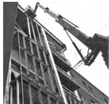
▲ Installation of a new stick-built curtain wall.
