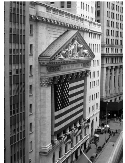
A New York Stock Exchange in New York, New York. Facility-Wide Roof Condition Assessment and Repairs.
