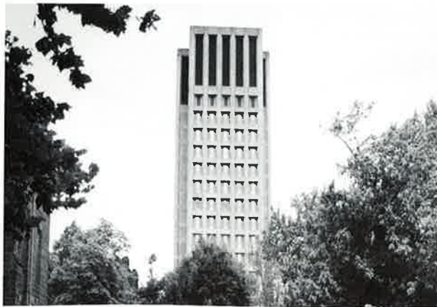
Kline Biology Tower at Yale University, New Haven, Connecticut.
