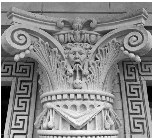
▲ The coating on this decorative terra cotta element protects the surface from exposure.
