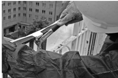
▲ Removal of a failed coating.
