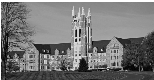
▲ Saint Thomas Seminary in Bloomfield, Connecticut. Bell Tower Facade Rehabilitation with Limestone Coating Replacement.
