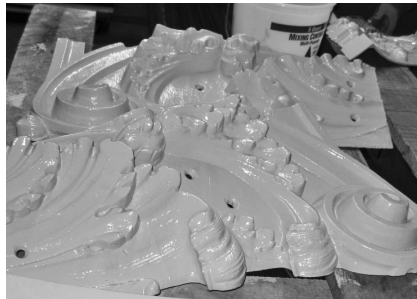
▲ Restoration and recoating of this cast iron element required off-site conservation.
