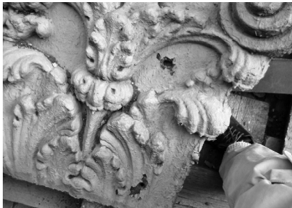
▲ Restoration and recoating of this cast iron element required off-site conservation.
