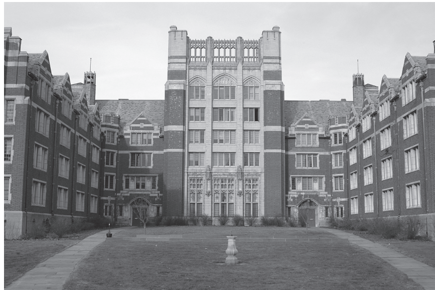
▲ Wellesley College, Tower Court (pictured), Severance Hall and Clafin Hall in Wellesley, Massachusetts. Slate Roof Replacement and Building Envelope Rehabilitation
