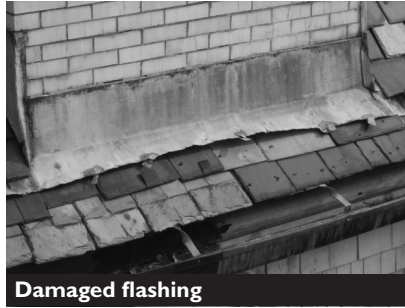
Damaged flashing
