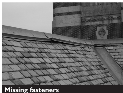
Missing fasteners
