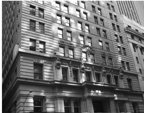
A Broad Exchange Building, 25 Broad Street in New York, New York. Landmark Terra Cotta Facade Restoration.
