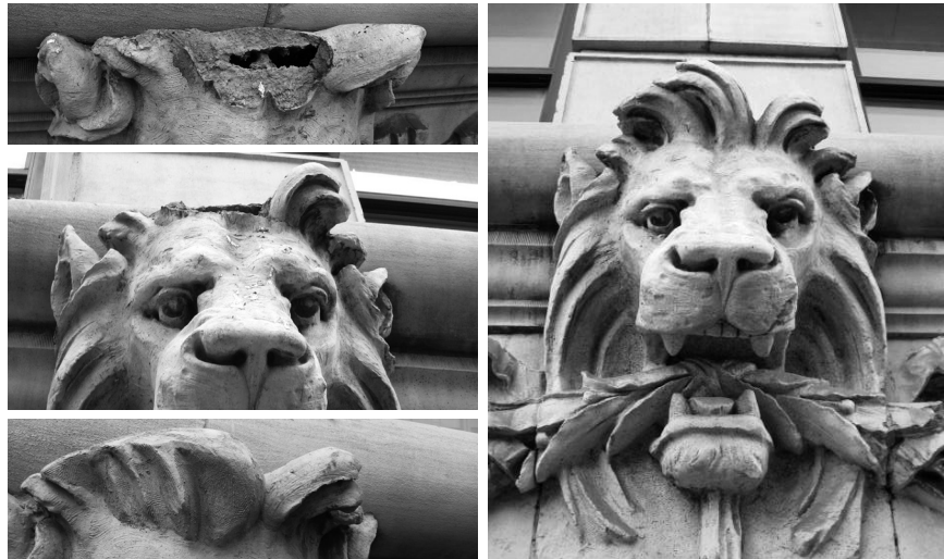
▲ Restoration of spalled terra cotta decorative element.
