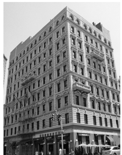
A Hotel Wales in New York, New York. Landmark Terra Cotta Repair and Replacement.
