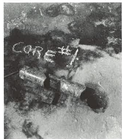
core showing subsurface cracking
