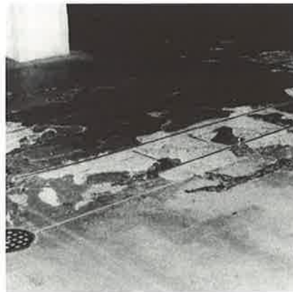
exposed reinforcement
