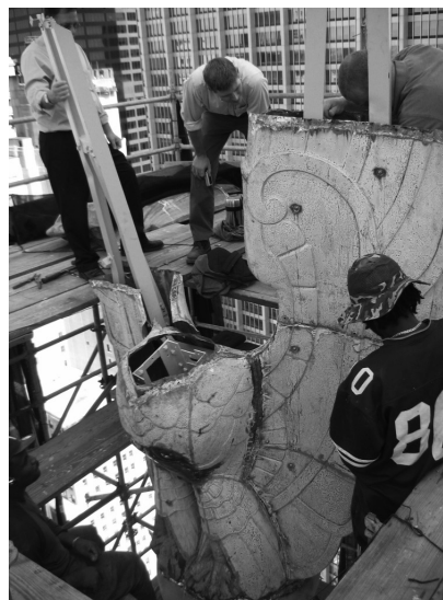
▲ Beyond roofing, copper is also used for ornamentation. Restoration of this copper eagle atop a 1929 high-rise involved off-site and on-site repair, cleaning, and reconstruction.
