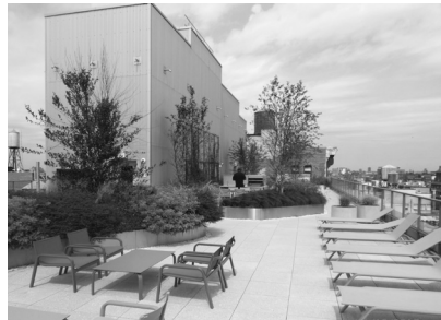
7W21 Flatiron Luxury Apartments in New York, New York. Building Envelope Consultation for Zinc Wall and Roof Systems.
