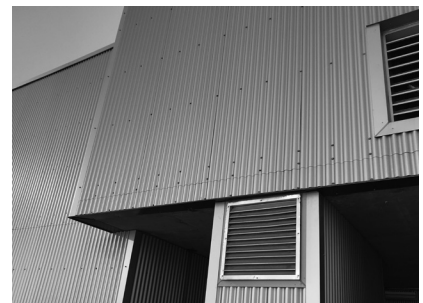
▲ A zinc facade system gives this rooftop mechanical room a sleek, modern look.
