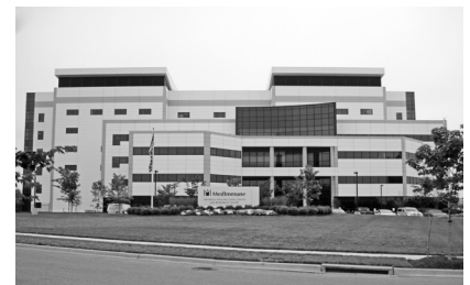
MedImmune Manufacturing Center in Frederick, Maryland. Leak Investigation at Coated Insulated Steel Panel Facade.
