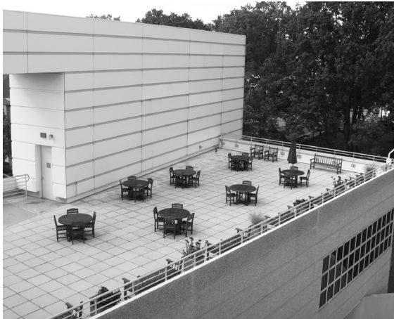
▲ Once considered budget cladding consigned to warehouses and industrial facilities, today's metal panel systems are viable options even for high-end projects.
