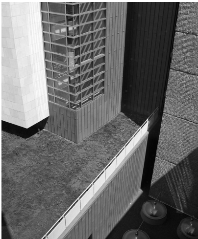
▲ Metal facade systems come in a variety of materials, including aluminum, copper, stainless steel, and zinc, pictured here.
