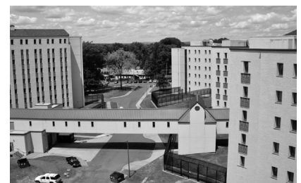
Rockland Psychiatric Center in Orangeburg, New York. Ice Buildup Mitigation at Metal Standing-Seam and Clay Tile Roofs.
