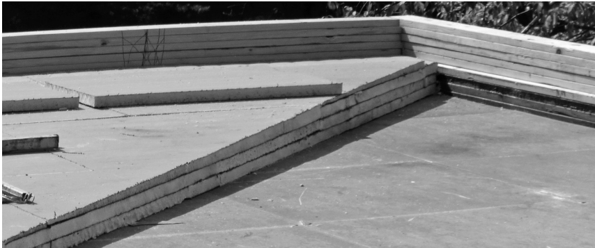
▲ When adding insulation to the roof, consider the impact on edges, terminations, and transitions, which may need to be adjusted to accommodate the additional depth.
