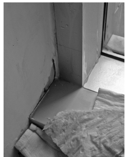
▲ New high-performance windows installed adjacent to conductive wall assemblies can still lead to condensation and moisture damage.
