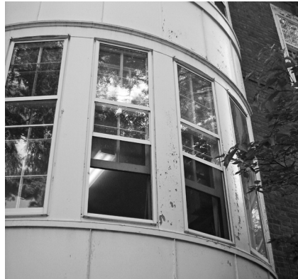
▲ High-performance replacement windows ( right ) resolve thermal inefficiencies and leaks that the retrofitted storm windows ( left ) at this historic building failed to adequately address.
