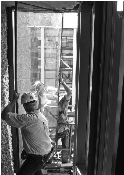
▲ Insulating glazing may be heavier than the original glass, requiring additional support.
