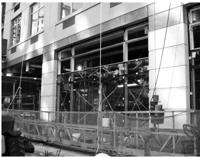
▲ Building codes specify glazing requirements for solar heat gain and thermal transfer.
