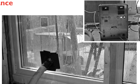
▲ On-site air and water leakage testing can provide a quantitative measure of in-situ window performance.
