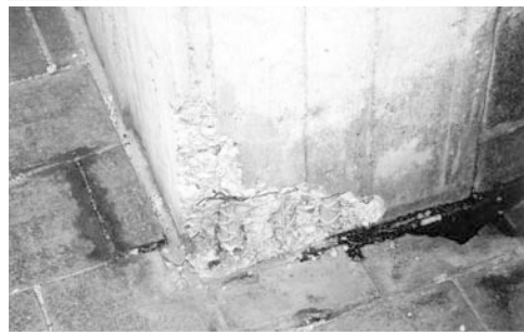
V Clockwise from bottom: Cracks at base of concrete column; spalled concrete and exposed steel reinforcement; severe deterioration at column base.
