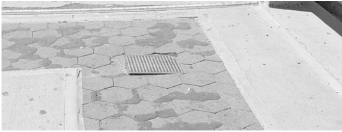
A Clockwise from above: Misaligned drain and oozing asphalt setting bed material make for a hazardous and unsightly wearing surface; deterioration at expansion joint; and, at joint between paved and poured wearing surfaces.
