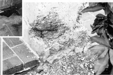
V Clockwise from bottom: Cracks at base of concrete column; spalled concrete and exposed steel reinforcement; severe deterioration at column base.
