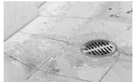
▲ Scaled concrete at drain may be indicative of standing water or inadequate drainage.
