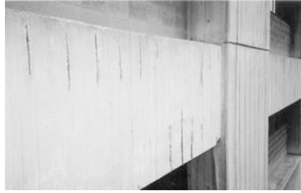
A Above left: Cracking and spalling of concrete panels on an exterior wall. Above right: Corrosion of embedded steel reinforcement has caused severe spalling at this corner.
