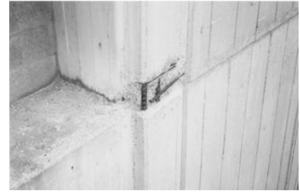
A Above left: Cracking and spalling of concrete panels on an exterior wall. Above right: Corrosion of embedded steel reinforcement has caused severe spalling at this corner.
