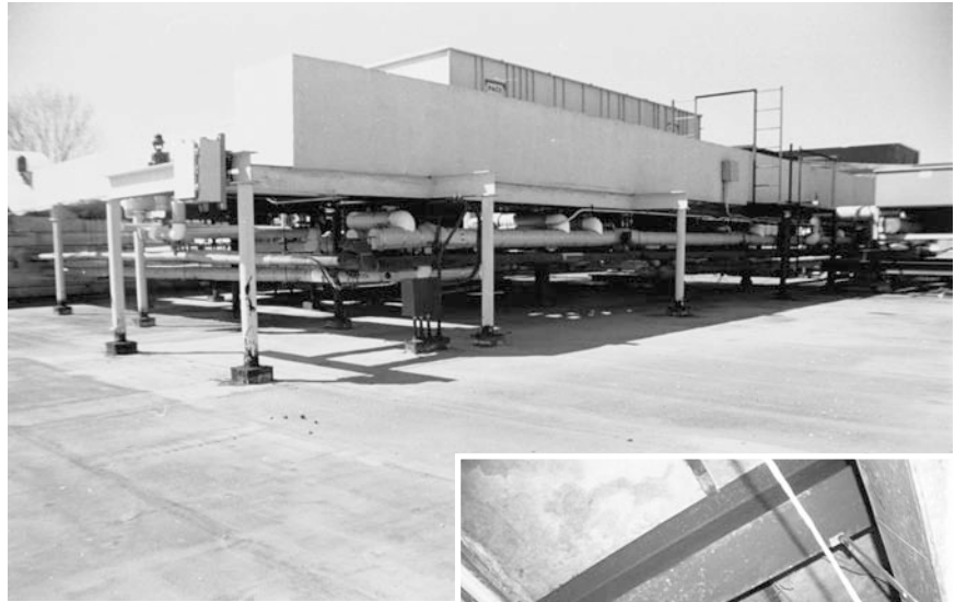
▲ What may seem like minor deterioration at the surface of this EPDM roof (above) has resulted in significant deterioration to the underside of the roof deck (shown at right) viewed from the interior:
