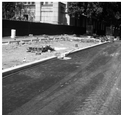
▲ Asphalt setting bed, ready to receive hexagonal asphalt pavers.
