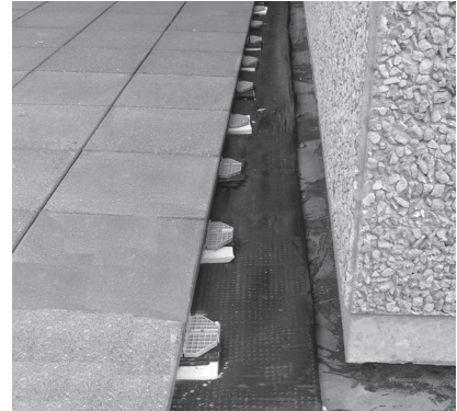
▲ Installation of a paver-on-pedestal system. Pavers are supported only at corners, with fully open joints.
