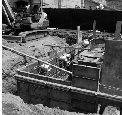
▲ Construction of concrete retaining walls.
