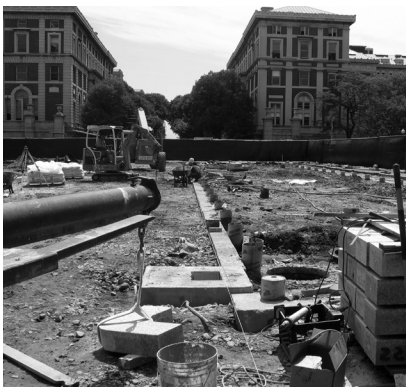
▲ Installation of granite curbs.
