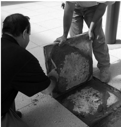
▲ Plaza investigation by an experienced architect or engineer uncovers the causes of water damage or deterioration.
