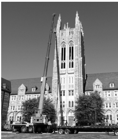
▲ Close-up investigation may be aided by lifts, drops, or other observation platforms.
