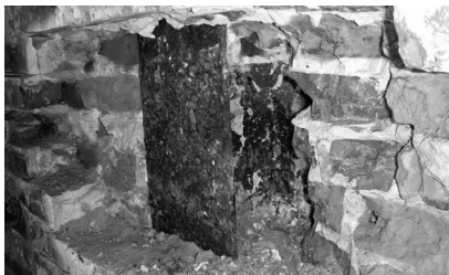
▲ Invasive probes can reveal concealed problems, such as corroded structural steel.
