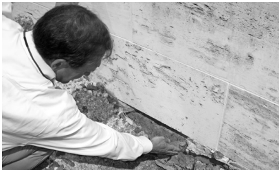
▲ Visual assessment permits close observation of defects at exterior walls.
