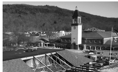
▲ Quinnipiac University in Hamden, Connecticut. Roof Assessment of 54 Buildings.
