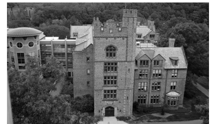
▲ Mount Holyoke College in South Hadley, Massachusetts. Assessment of 20 Buildings.
