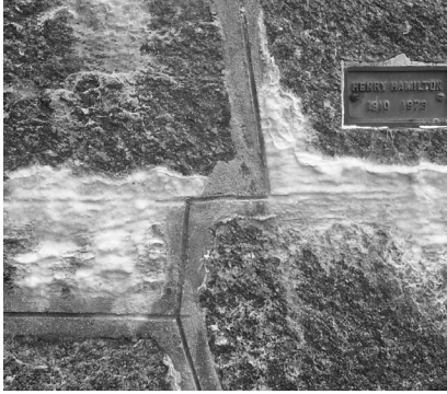
▲ Efflorescence.
