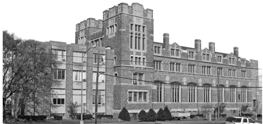
▲ Father O'Connell Hall at The Catholic University of America in Washington, District of Columbia. Limestone and Granite Facade Investigation and Restoration.
