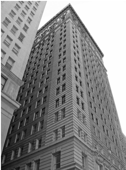
A Broad Exchange Building (1902) in New York, New York. Window Study and Restoration Design.
