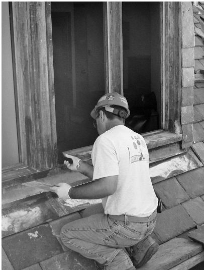
▲ A carpenter restores wood window casing using epoxy repair materials.
