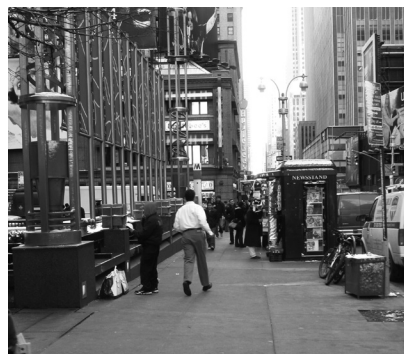
▲ Paramount Plaza, New York, New York, Pedestrian Tunnel Leak Investigation.
