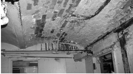
▲ At street level ( top left ), the sidewalk appears to be in good condition. In the vault below ( bottom left ), masonry arches show their age but seem structurally stable. Masonry removal, however, shows how badly deteriorated the embedded steel really can be ( above ).
