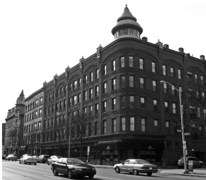
▲ One Linden Place, Hartford, Connecticut, Electrical/Boiler Room Vault Rehabilitation.
