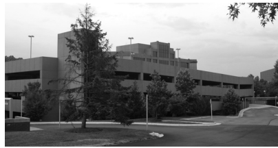
West*Park Garages in McLean, VA. Investigation of Four Garages.
