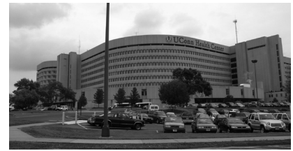
University of Connecticut Health Center in Farmington, CT. Garage Assessment.
