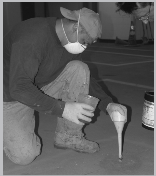
▲ Above: Test core showing epoxy penetration to the bottom of a crack.
