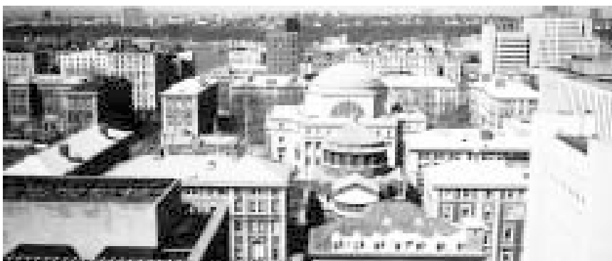
▲ Columbia University Morningside Campus, 60 Buildings. Facade and Roof Investigation and Rehabilitation.
