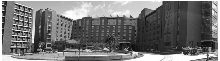
University of Connecticut, NextGen Hall Dormitory , Storrs, Connecticut, Building Envelope Consultation.
