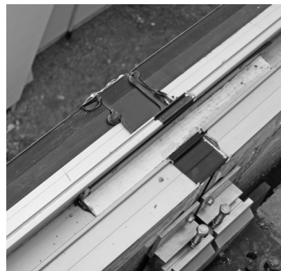
Curtain wall installation review: Creating a water-tight intersection is a multi-step process, beginning with application of sealant at the glazing pocket ( left ), then placement of metal covering over the gap ( center ), followed by appropriate tooling of sealant at the horizontal weather seal ( right ).
