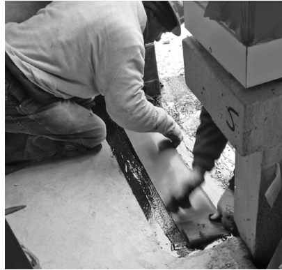
Waterproofing installation review: As potential sources of water infiltration, thresholds demand attention to detail. Here, asphalt and roofing felt ( left ) are applied under the flashing membrane ( center ) to create a positive lap, then the roofing base membrane is embedded into the asphalt ( right ).
