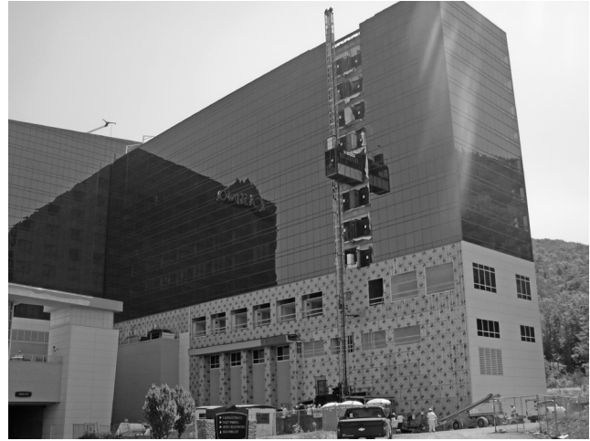
Curtain wall construction at this glass high-rise involved quality control of fabrication, assembly, installation, and field verification, to see that the final product meets design standards for performance and sustainability.
