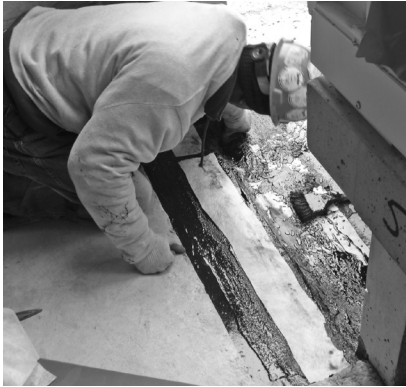
Waterproofing installation review: As potential sources of water infiltration, thresholds demand attention to detail. Here, asphalt and roofing felt ( left ) are applied under the flashing membrane ( center ) to create a positive lap, then the roofing base membrane is embedded into the asphalt ( right ).
