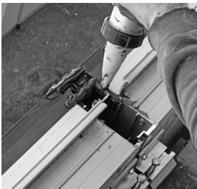
Curtain wall installation review: Creating a water-tight intersection is a multi-step process, beginning with application of sealant at the glazing pocket ( left ), then placement of metal covering over the gap ( center ), followed by appropriate tooling of sealant at the horizontal weather seal ( right ).
