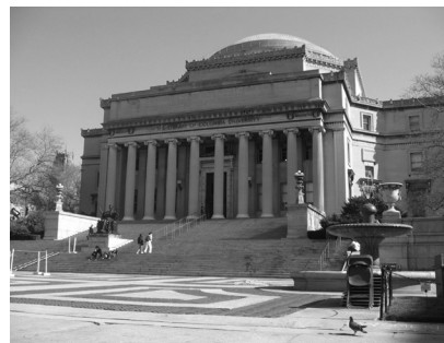
▲ Low Memorial Library at Columbia University in New York, NY. Roof Replacement.
