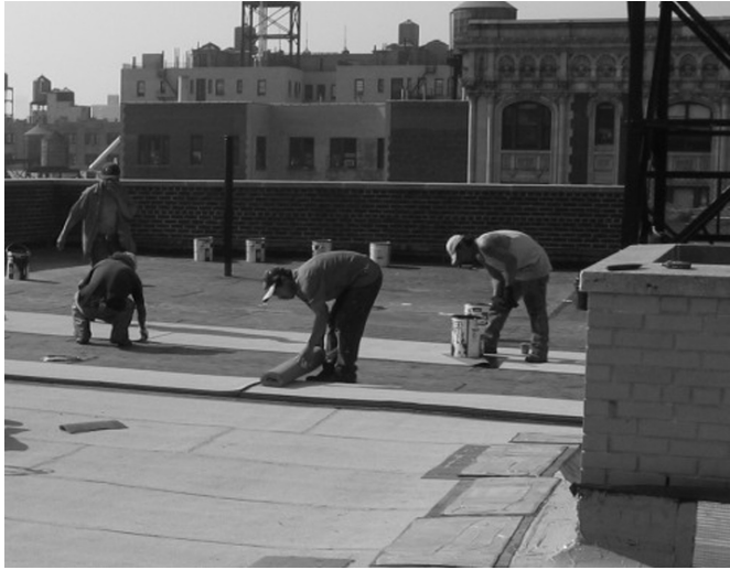
▲ Some cold-applied MBRs offer a simple, “peel-and-stick” installation that minimizes the chance of installer error.
