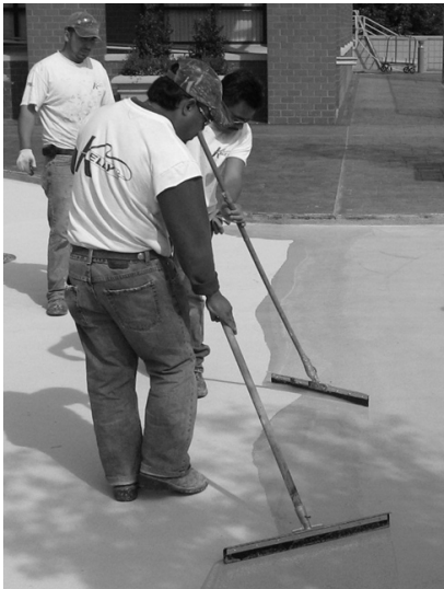
▲ Liquid-applied roofing membranes offer easy application, with no bulky rolls or open flames to negotiate.
