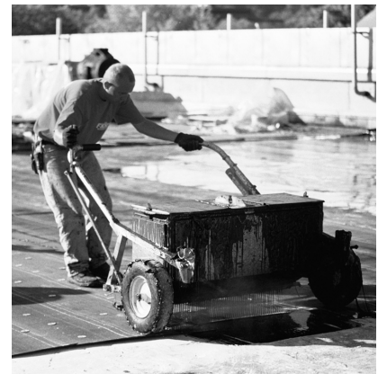
■ Torch-applied ( left ) and cold-applied MBRs (see photo on page 4 ) provide the resilience and durability of traditional built-up systems, without the need of lifting or pumping 400°F molten asphalt onto the roof ( above ).
