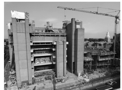
▲ Art and Architecture Building at Yale University in New Haven, CT. Building Envelope Rehabilitation, including Roof Replacement.
