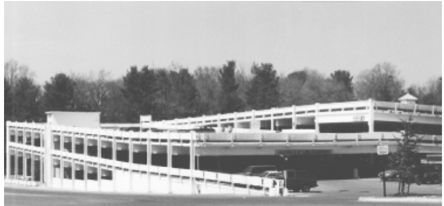
▲ Bishops Corner Parking Facility West Hartford, Connecticut (Edens & Avant)
