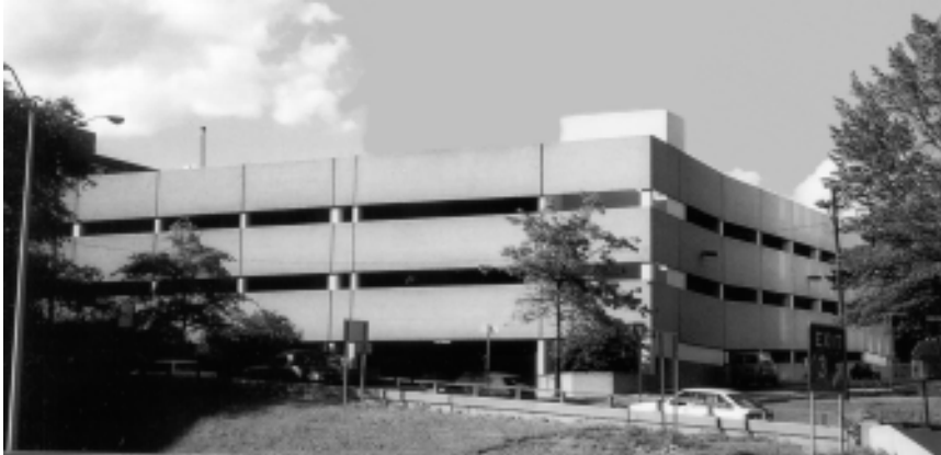
▲ SNET's George Street Garage New Haven, Connecticut (Southern New England Telephone Company)
