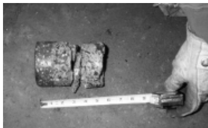
▲ Concrete core has been extracted from a parking deck for analysis.
