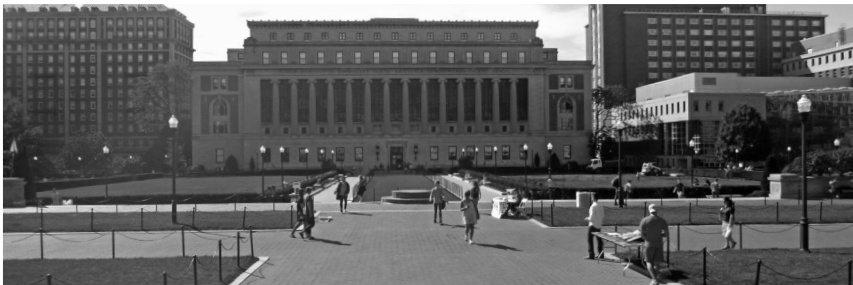
▲ Columbia University, Butler Library , New York, New York, Plaza and Hardscape Rehabilitation.
