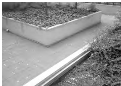
▲ Plaza spaces require continuous waterproofing protection, including installation of membranes in planters and on vertical surfaces.
