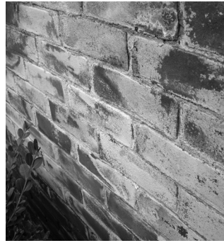
▲ Efflorescence.
