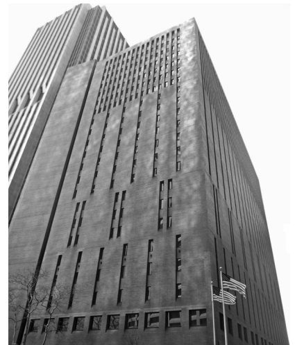
▲ Edge Fund Advisors, 4 New York Plaza in New York, New York. Facade Investigation and Rehabilitation.
