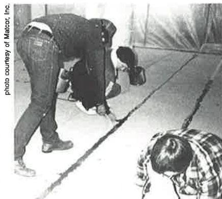
installing anode material in cathodic protection system
