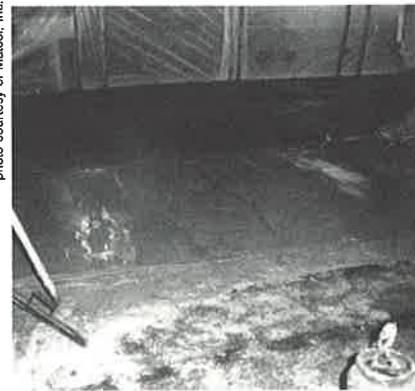
installing wearing surface over anode
