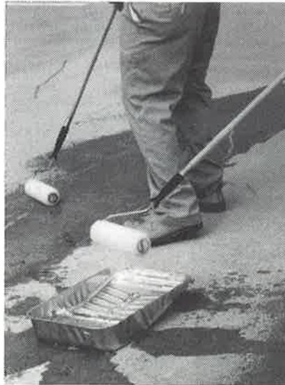
installing sealer - note darkening of concrete
