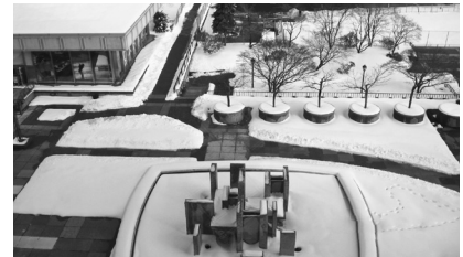
▲ Constitution Plaza in Hartford, Connecticut. Plaza, Garage, and Exterior Stair Rehabilitation.
