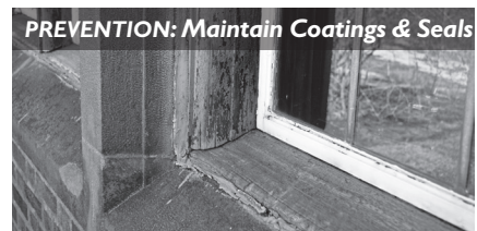
Freeze-Thaw and Salt Damage
