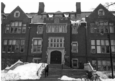
▲ Mount Holyoke College in South Hadley, Massachusetts. Exterior Envelope Assessment of 20 Buildings.
