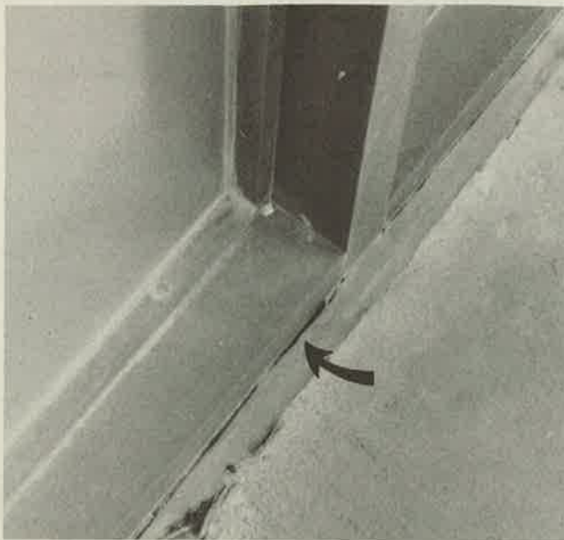
Adhesive Failure
