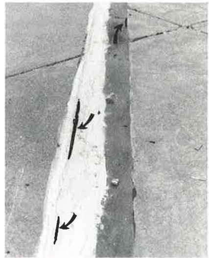
adhesive failure
