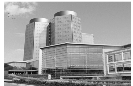
▲ Stony Brook University Medical Center, Stony Brook, New York, Curtain Wall Replacement (rendering).
