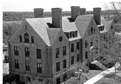
▲ Connecticut College, Fanning Hall, New London, Conn., Slate Roof Condition Survey.
