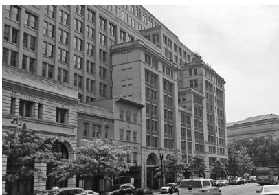
▲ 1001 Pennsylvania Ave., Washington, DC, Roof Terrace Surveys and Replacements.
