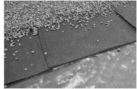
A In this vegetative roof above a parking garage, insufficient drainage caused ponded water (left). The new assembly (right) incorporates waterproofing membrane, drainage mat, and gravel.
