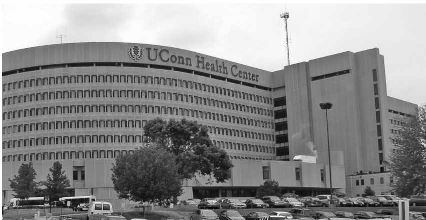
▲ University of Connecticut Health Center in Farmington, Connecticut. Facade Sealant Replacement.
