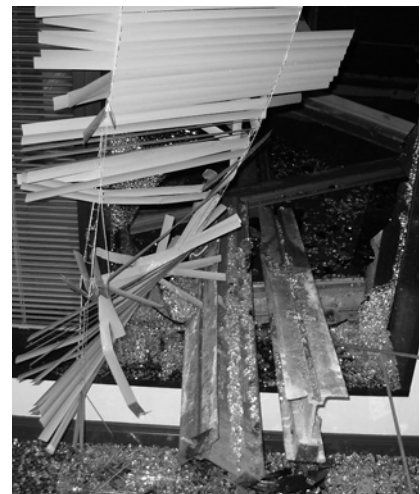
A In high winds, these steel beams became dangerous projectiles.
