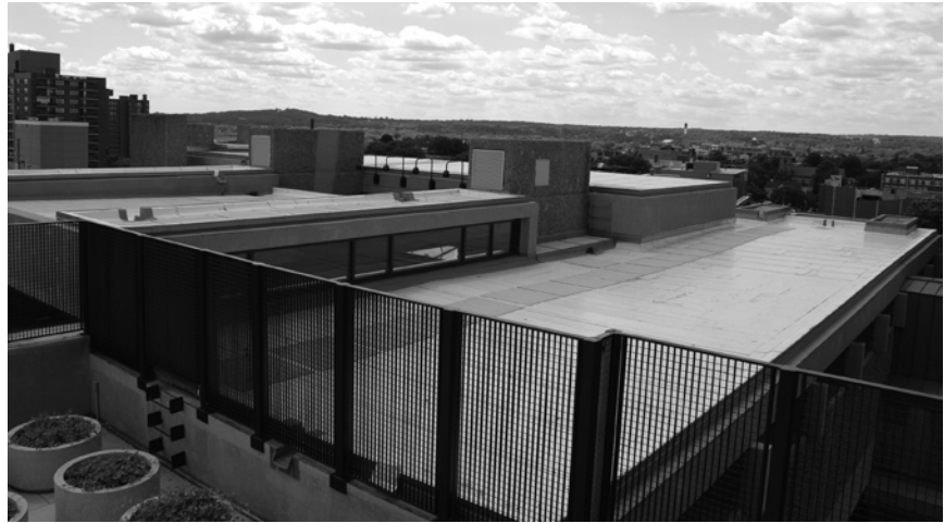
▲ Cool roofs reflect heat, cutting energy costs and normalizing urban temperatures. Pictured here is a modified bitumen roof (MBR) with a reflective capsheet.
