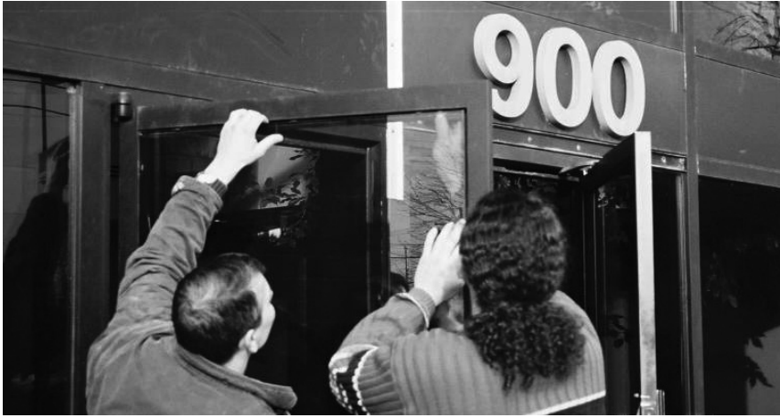
▲ Poorly performing doors make HVAC systems work overtime to stabilize temperature.
