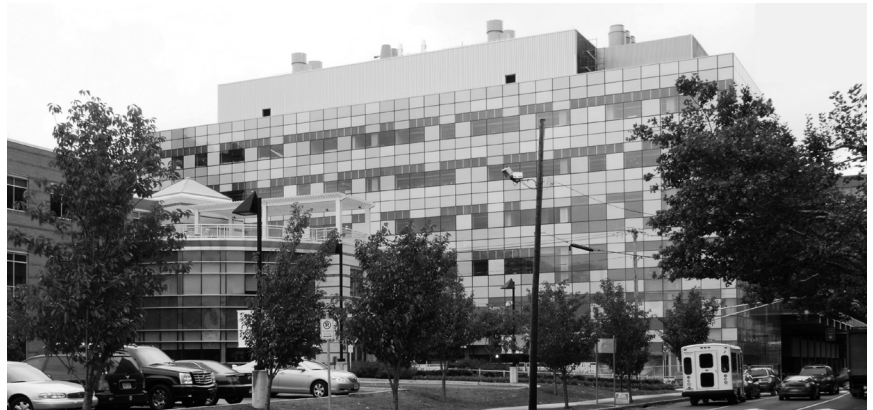
▲ Yale-New Haven Hospital, 55 Park Street Laboratory in New Haven, CT. New construction consultation and feasibility assessment for curtain wall, roofing, and foundation waterproofing.
