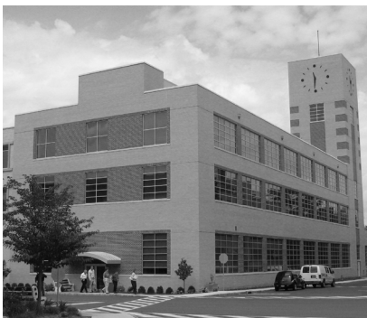
▲ Schering-Plough Corporation in Summit, NJ. Facade reconstruction to improve energy profile and aesthetics. New Jersey Golden Trowel Award, Special Recognition.
