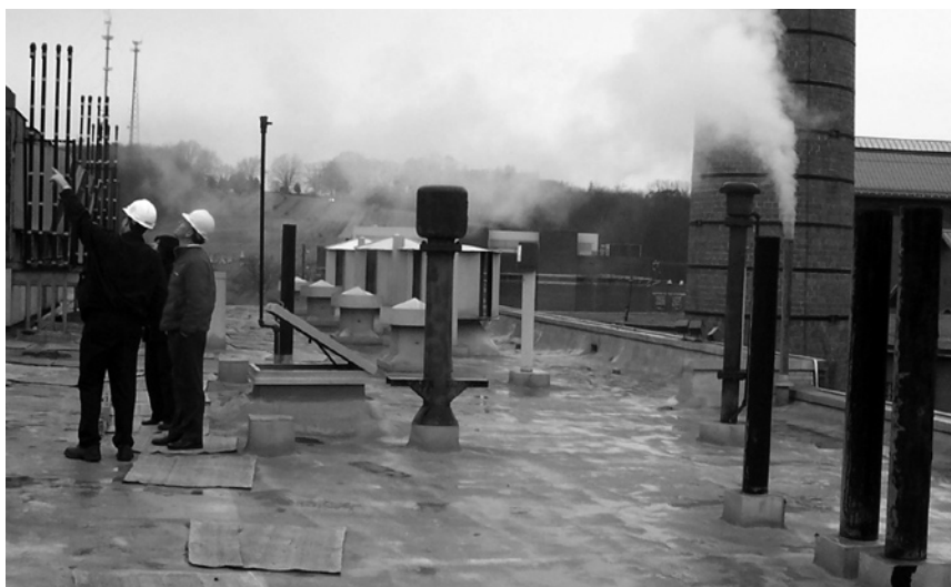
▲ As the barrier between the indoor and outdoor environments, the building envelope is critical to energy performance.
