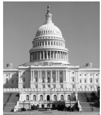
▲ United States Capitol Building in Washington, District of Columbia. Water Penetration Study and Dome Restoration that received the AIA New England Regional Council Design Award
