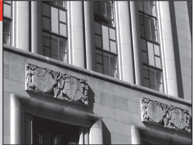
▲ Refurbishing, rather than replacing, older buildings saves energy and materials. Here, restoring steel windows preserved historic character while minimizing costs and ecological impact.
