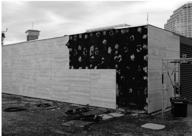
▲ Penthouse marble panel replacement in process.
