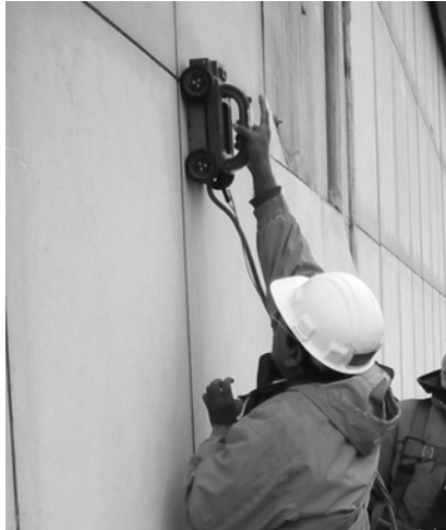
▲ Ground-Penetrating Radar (GPR) identifies anchor locations without removing panels.
