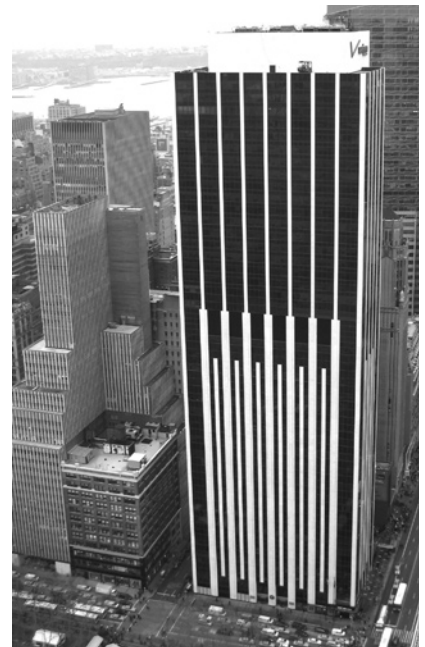
Corporate High-Rise at 1095 Avenue of the Americas in New York, New York. Marble and Glass Curtain Wall Consultation.
