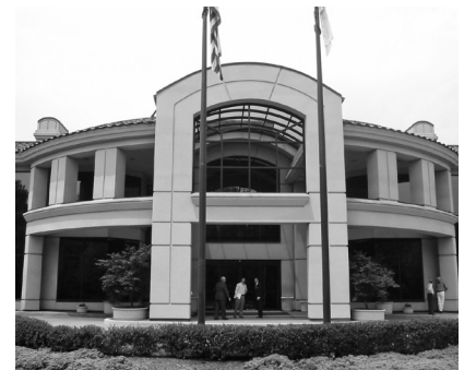
▲ Pfizer, Inc., North Maple Inn in Basking Ridge, New Jersey. Facade Rehabilitation.
