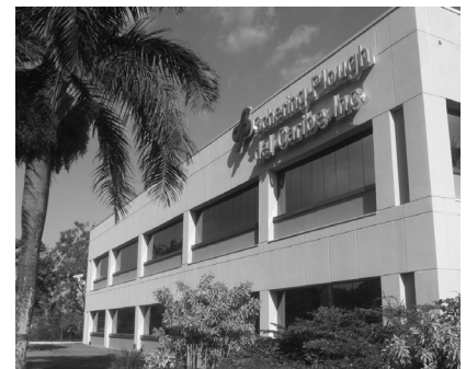
▲ Schering-Plough del Caribe in Toa Baja, Puerto Rico. Facade Reconstruction.
