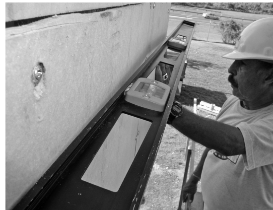
▲ To true the wall surface, the installer should level the insulation board, rather than build up base coat.
