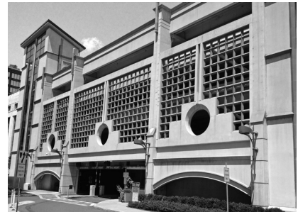
▲ State University Construction Fund in Albany, New York. Garage Assessment/Repair.
