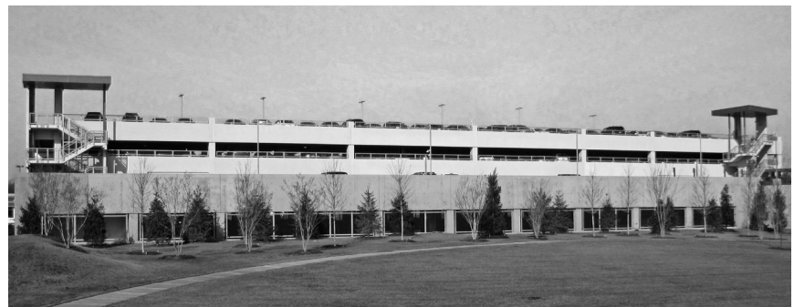
▲ Washington Gas Springfield Operations Center in Springfield, Virginia. Garage Assessment.
