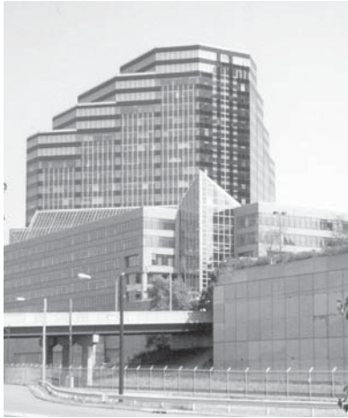
▲ Glass curtain wall and window systems at a suburban corporate office park.
