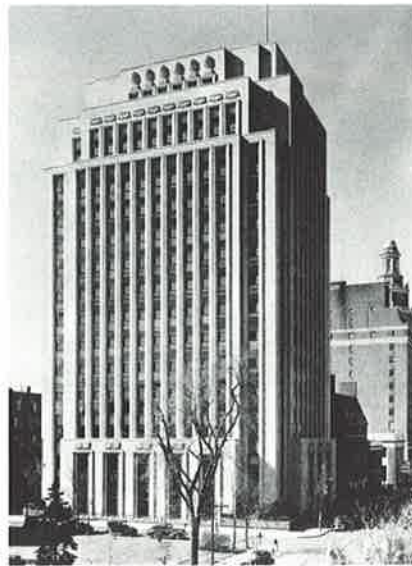
SNET Headquarters, New Haven CT. Photo courtesy of SNET
