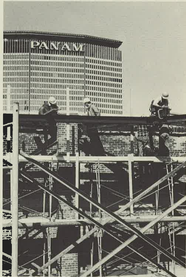
Field Representatives monitor construction
