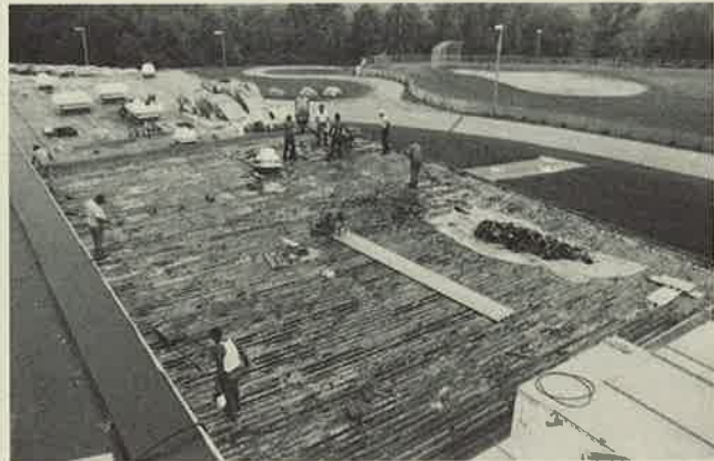
Reroofing Ridgefield High School. Ridgefield, CT
