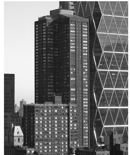
▲ The Sheffield in New York, New York. Window and Facade Water Testing.
