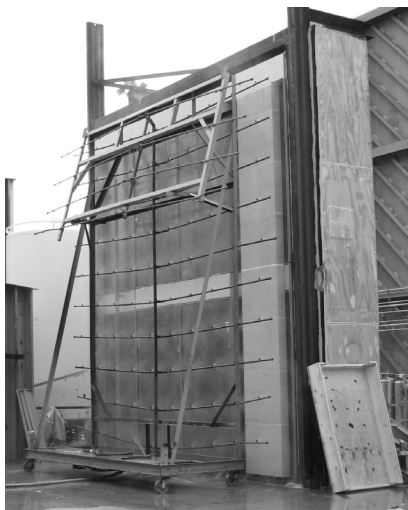
▲ Off-site spray rack testing allows the design professional to verify water-tightness of the proposed assembly.
