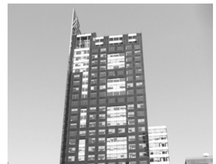
▲ Bertelsmann Building, 1540 Broadway in New York, New York. Glass Curtain Wall Investigation and Repair.
