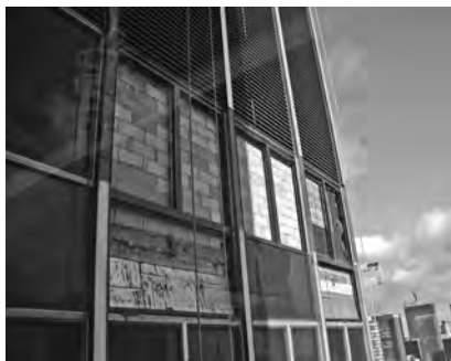
❑ Figures 8a (top), 8b (middle), 8c (bottom): A portion of this glazed curtain wall detached and fell dozens of stories.
