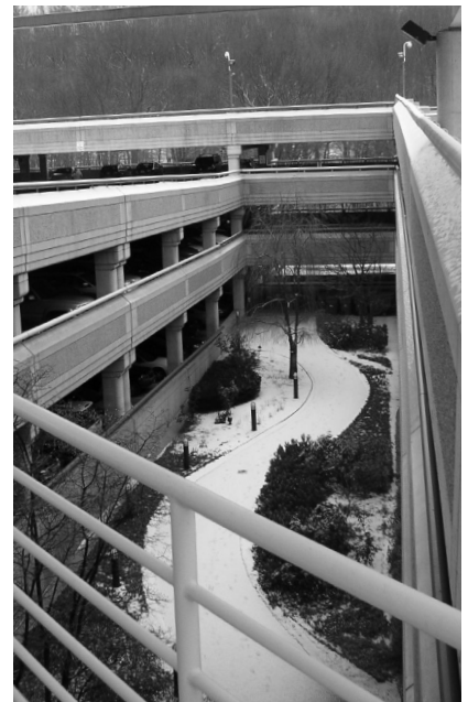
▲ Quinnipiac University, Anthem Campus in North Haven, Connecticut. Condition Evaluation.
