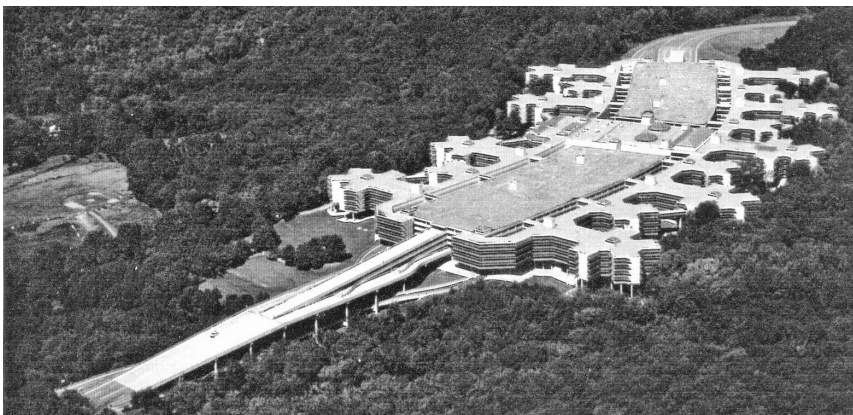
▲ The Corporate Center (former Union Carbide Headquarters) in Danbury, Connecticut designed by Kevin Roche (1982). Building Envelope and Garage Rehabilitation.
