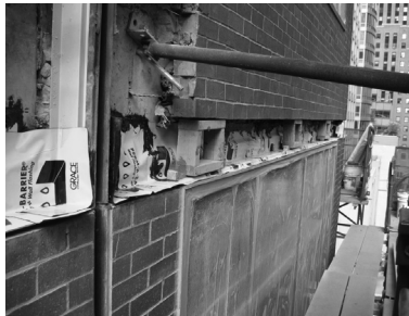
Installation of new flashing at window head.
