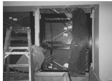
Installation of replacement windows.
