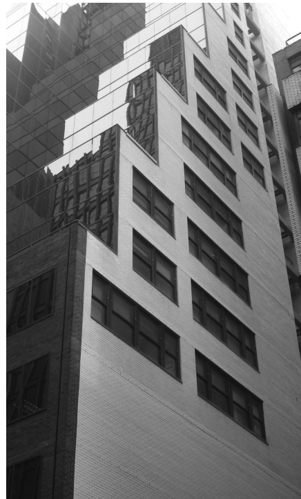
Reconstruction of brick exterior wall after flashing replacement.
