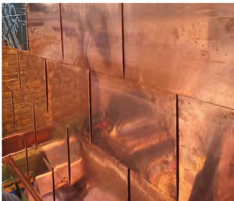
Overlapping copper sheet metal wall cladding with lock seam joints.
