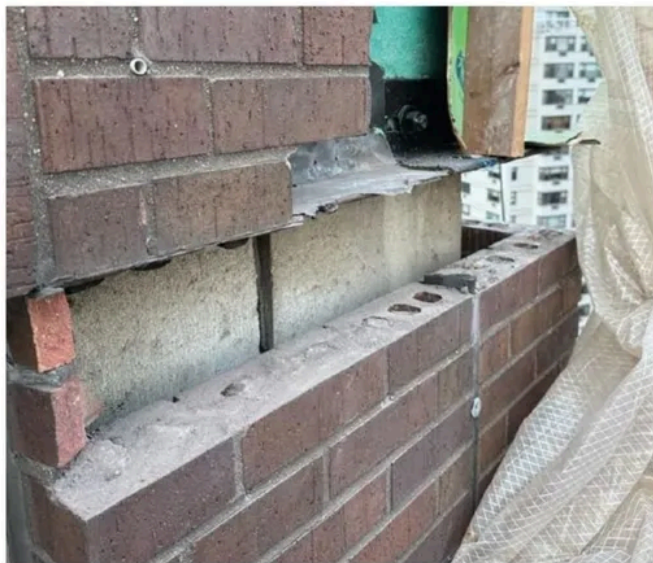
Pictured: water-proofing at masonry cavity wall relieving angle
