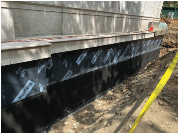
Left: Positive-side foundation waterproofing is applied to the exterior. Right: Negative-side waterproofing is on the interior.
